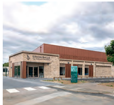
Build and Rebuild
